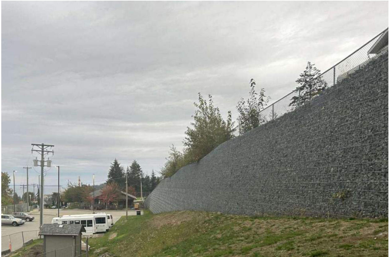
Photograph 5: View of the exposed retaining wall base, looking northwest
