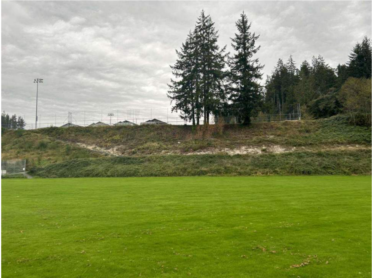
Photograph 1: Profile view of the fill slope, looking northwest.
