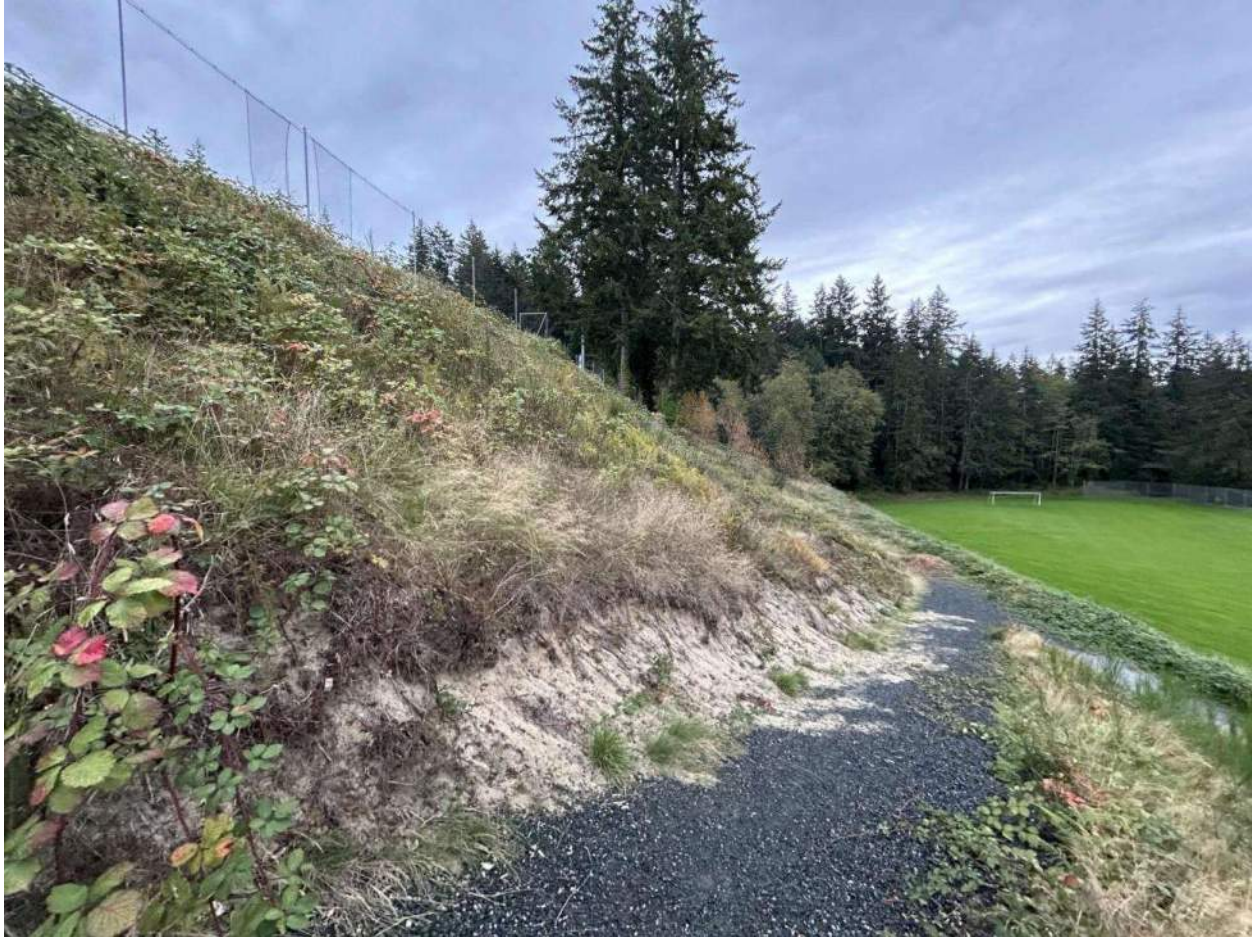
Photograph 3: View of the fill slope soil conditions, looking southeast.
