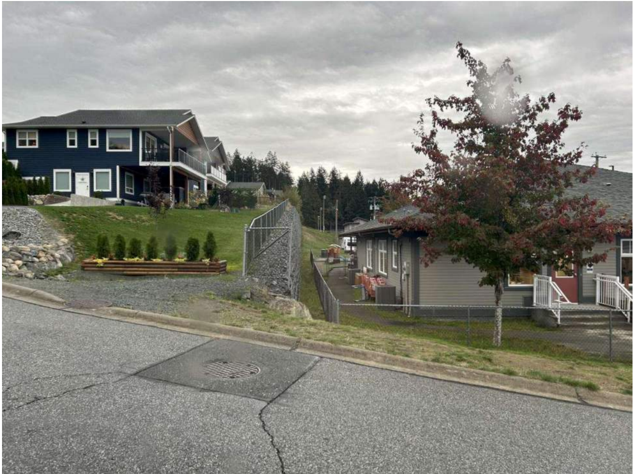
Photograph 6: Side view of the retaining wall and building offsets, looking southeast.
